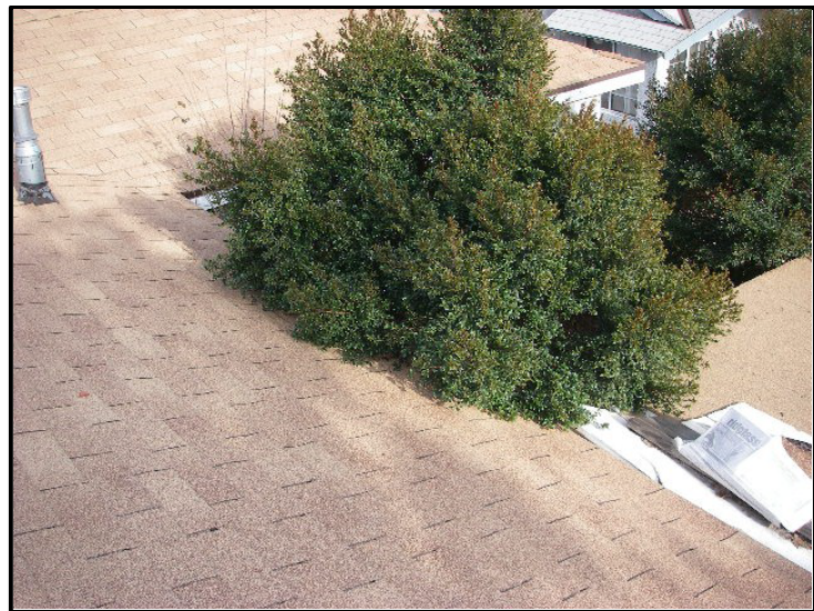
View of tree in contact with roof.
