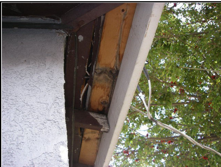
View of unpainted and water damaged wood at soffit and eave.
