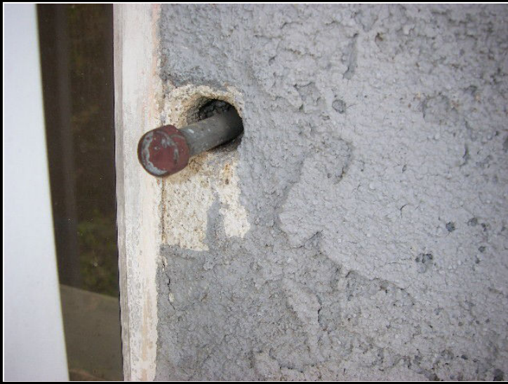
View of gap between pipe and wall, and missing stucco.
