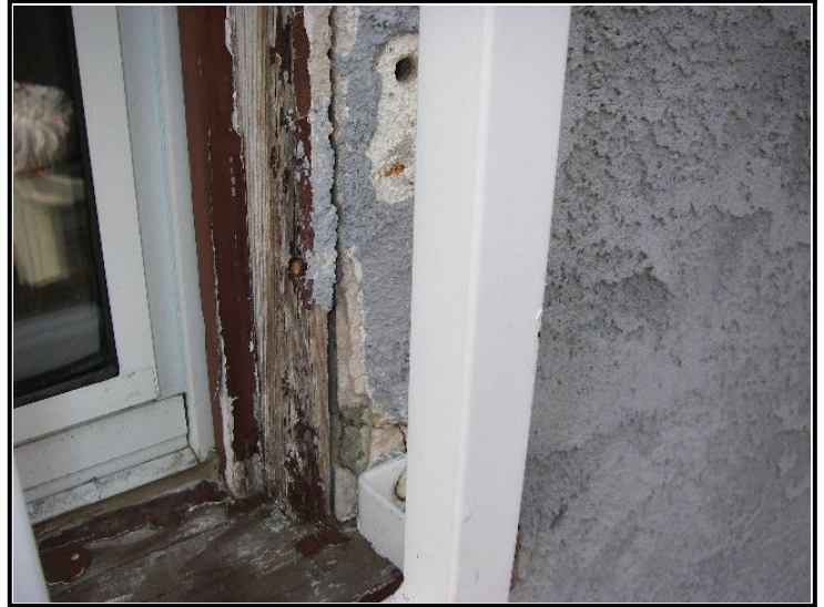
View of missing and peeling paint at window frame.
