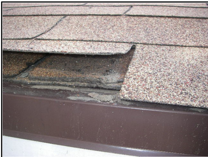
View of lifting shingle.
