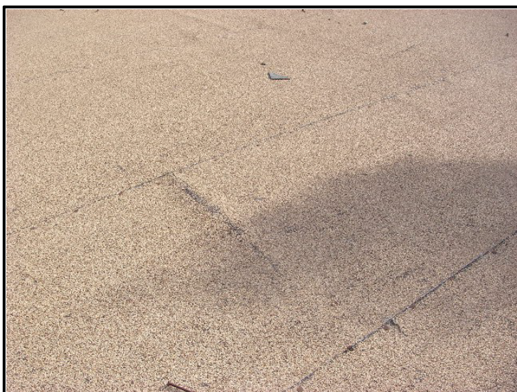
View of wrinkling and missing granules.
