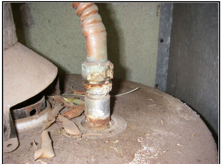
View of corrosion on plumbing.
